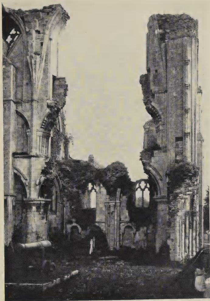
MALMSBURY, THE SHATTERED NAVE
